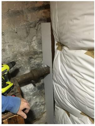
Some of the posts of the structure aren't quite vertical, requiring precision in cutting foam insulation:
